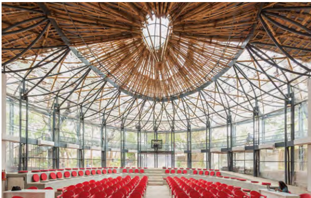
The Pavilion for the Kochi-Muziris Biennale 2018, 2018, Kochi, Kerala, India Premio Speciale L'Arca International: Anagram Architects per Kochi Biennale Foundation
