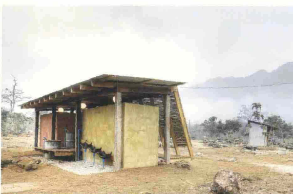
Premi Speciali Premio Speciale Stanislaw Niewo Client: Tasanee Keerepraneed Project: TYIN Tegnestue Title: Safe Haven Library and Safe Haven Bathhouse Construction: 2009, Ban Tha Song Yang (Tak), Thailandia
