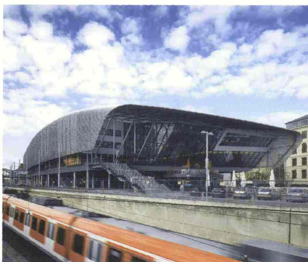
Premio Speciale Regione del Veneto Client: HOCHTIEF Projektentwicklung GmbH Project: Auer+Weber+Assoziierte Title: Central bus station Construction: 2009, Monaco (Bavaria), Germania
